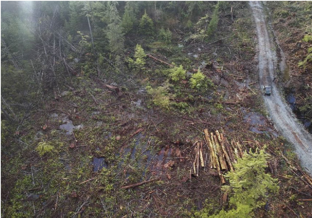
Island Timberland's puncheon road in a wetland on Read Island 55
